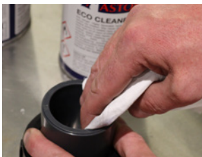
Clean pipe first
