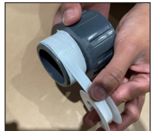
Take the threaded connector for the MPV. Wrap PTFE tape clockwise around the thread multiple times to ensure a water tight connection.
