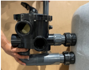
“Dry fit” pipework first
